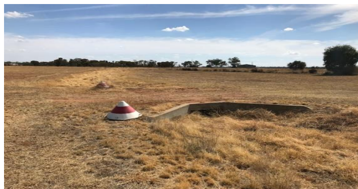
Photo 11: 7m wide culvert installed along proposed access road
